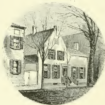
COLONIAL HOUSE, UNION STREET.
